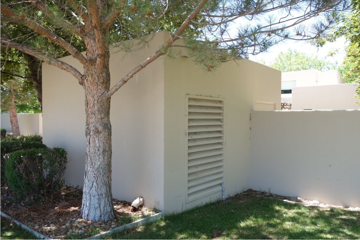
Visitor Center Storage Building - FCA Building #3813 Description: Exterior of the Building.
