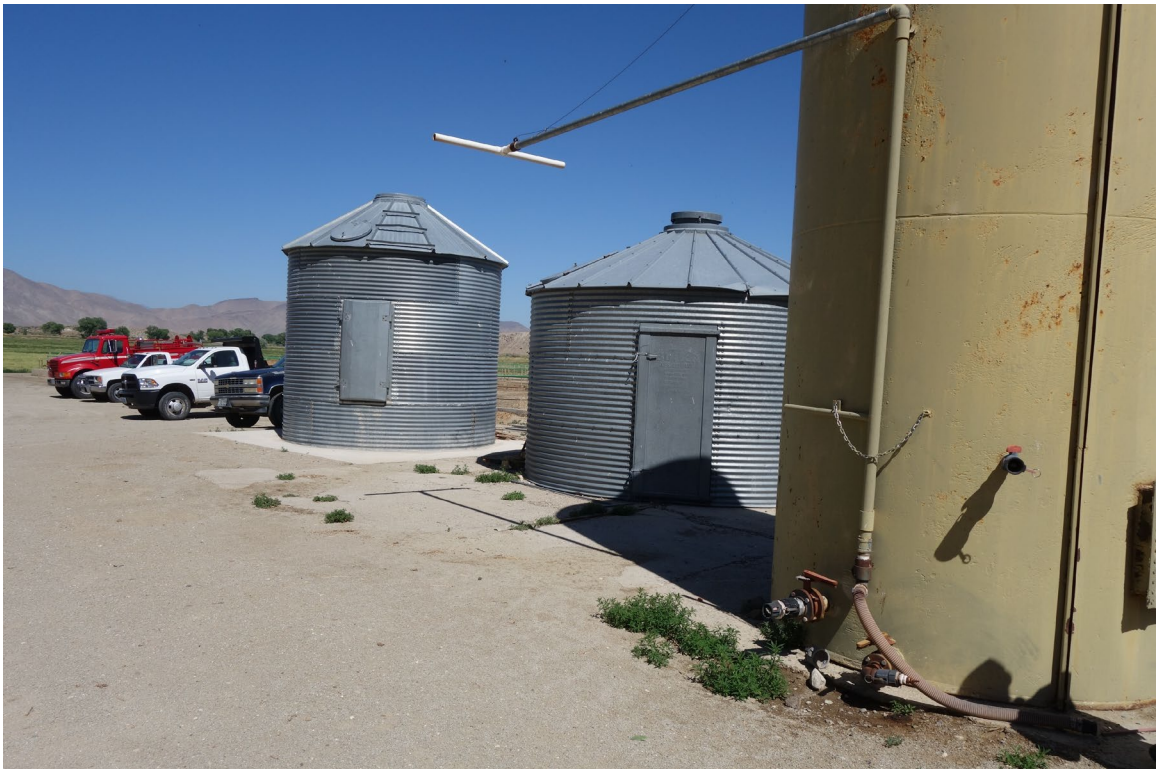
Silo 1, Silo 2 – FCA Building #3838, #3839 Description: Exterior of the Structures.
