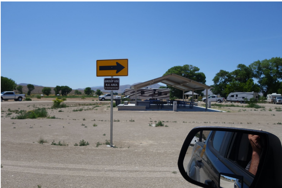
Group Use Ramada #2 – FCA Building #4048 Description: Exterior of the Building at Quail Run RV Camping Area.
