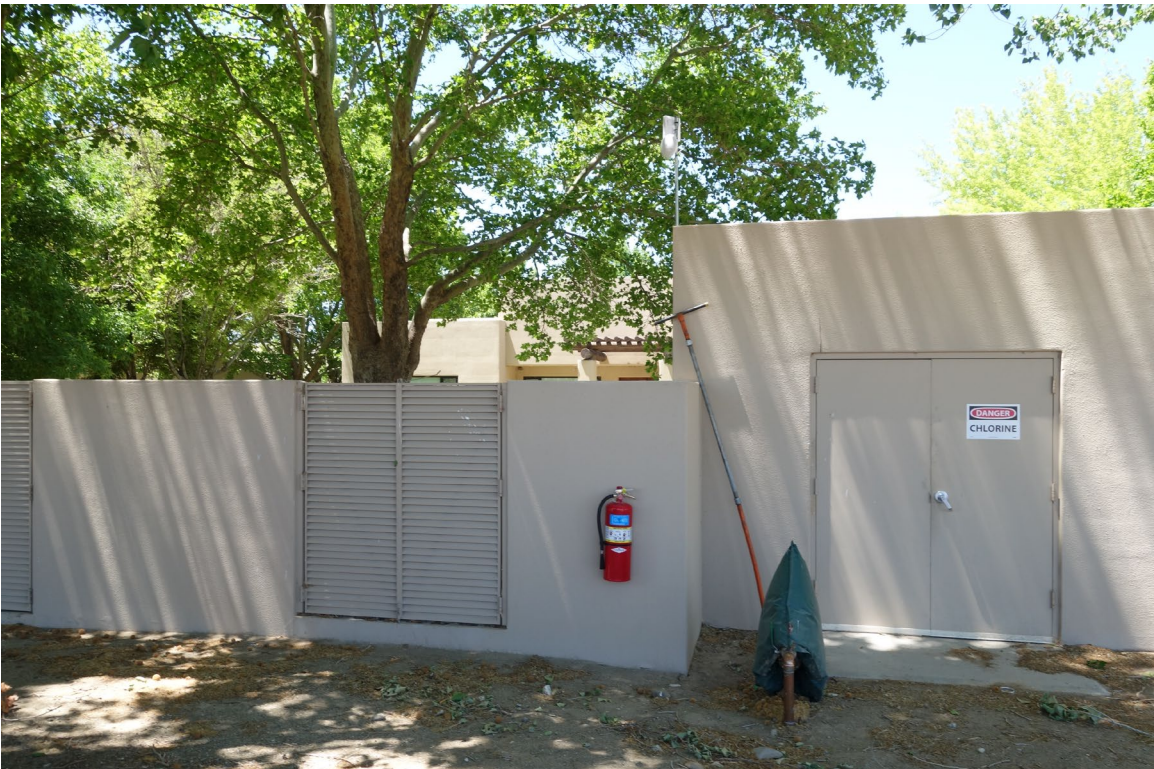
Guest House Domestic Well Building – FCA Building #3819 Description: Exterior of the Building.
