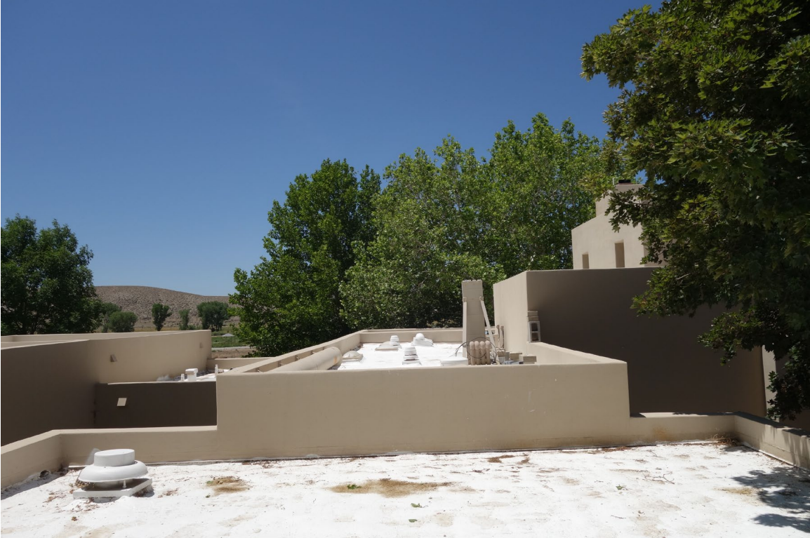
Visitor Center - FCA Building #3812 Description: Roof Repairs / Replacement Recommended.
