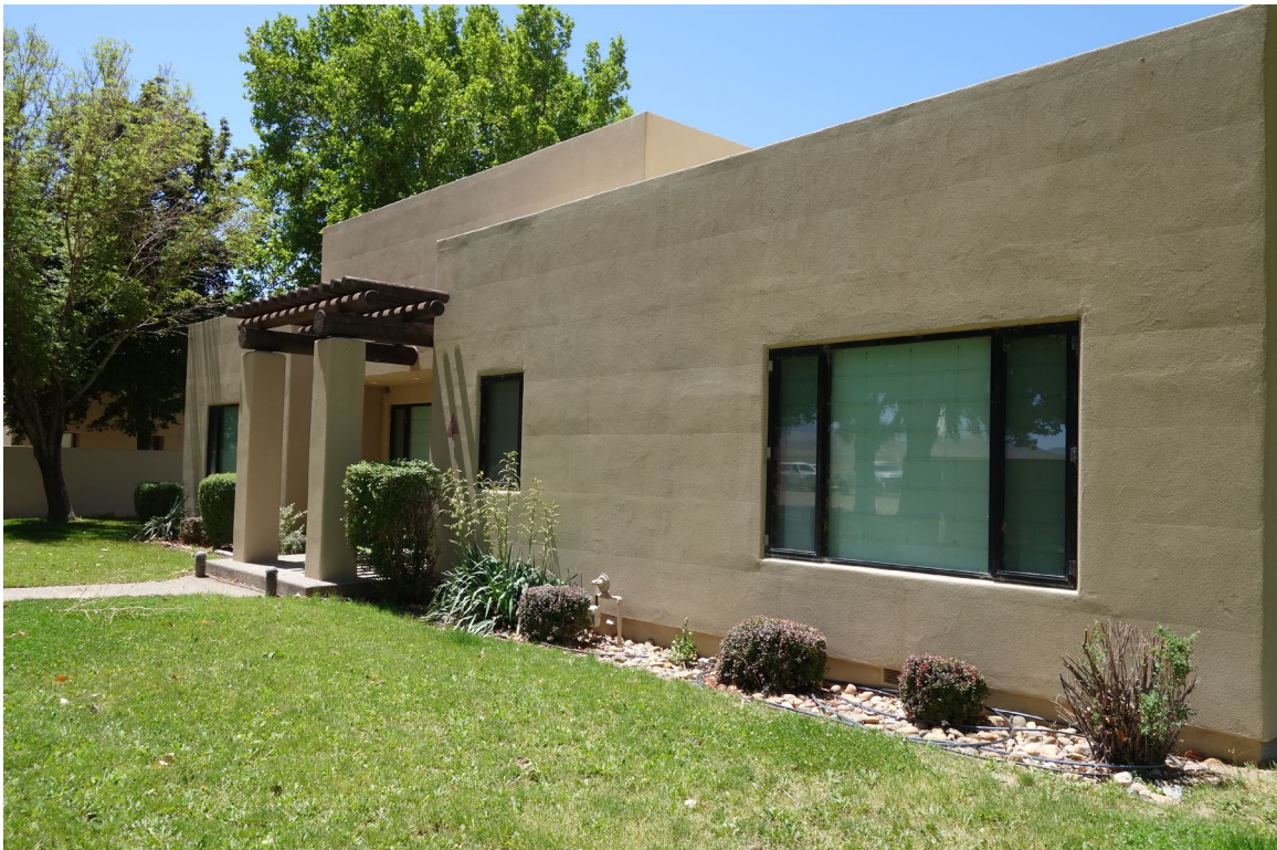
Guest House – FCA Building #3818 Description: Exterior of the Building.
