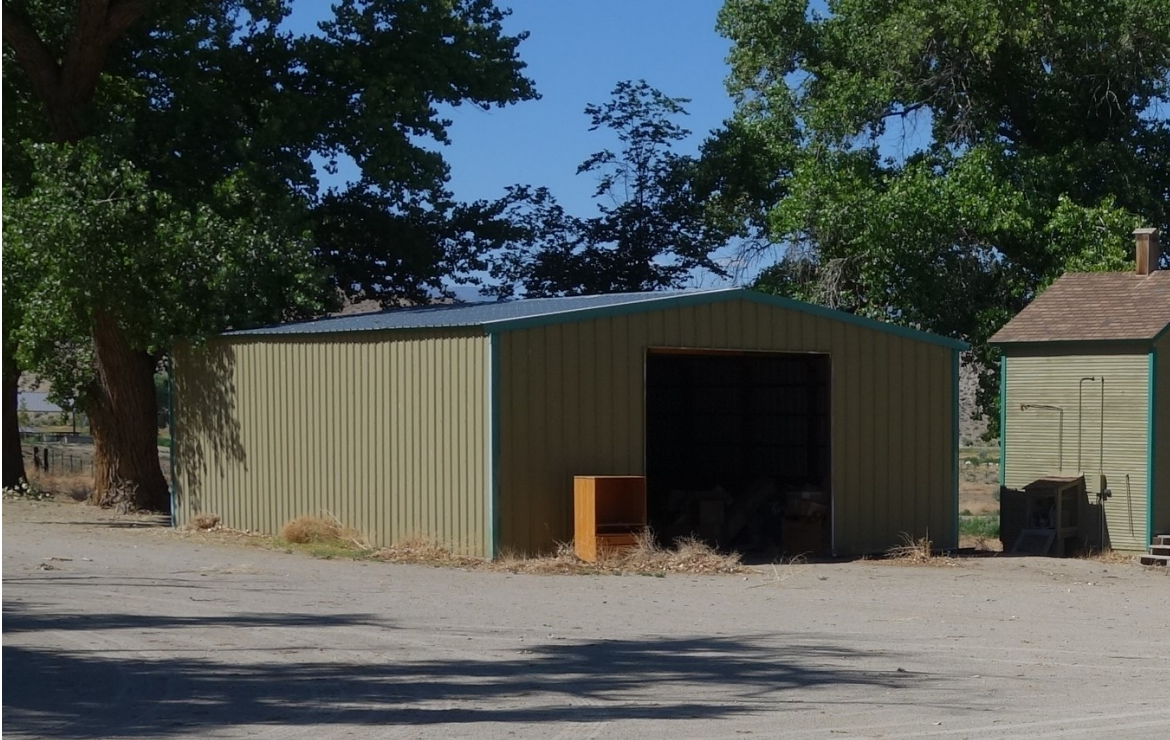
Church Shed – FCA Building #3830 Description: Exterior of the Building.
