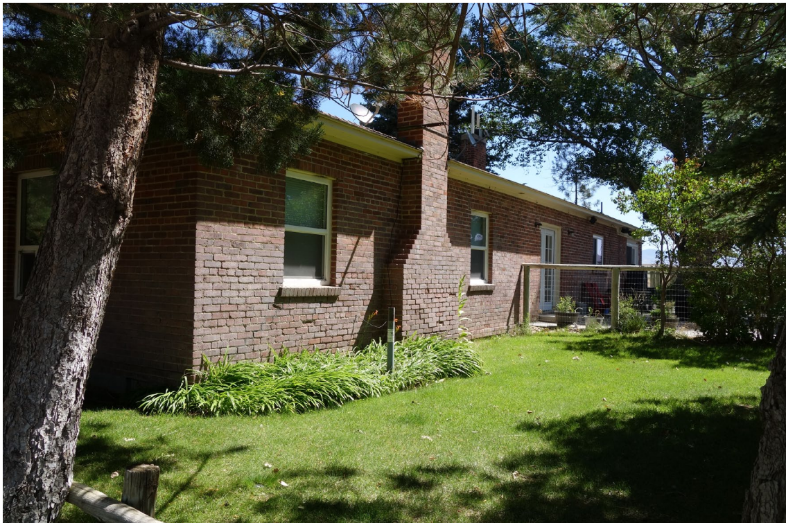
Brick House – FCA Building #3816 Description: Exterior of the Building.
