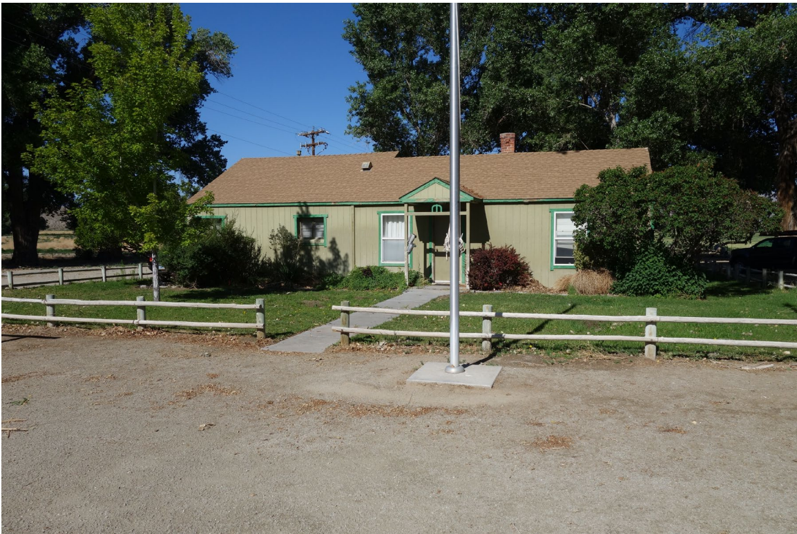
Chefs House – FCA Building #3822 Description: Exterior of the Building.
