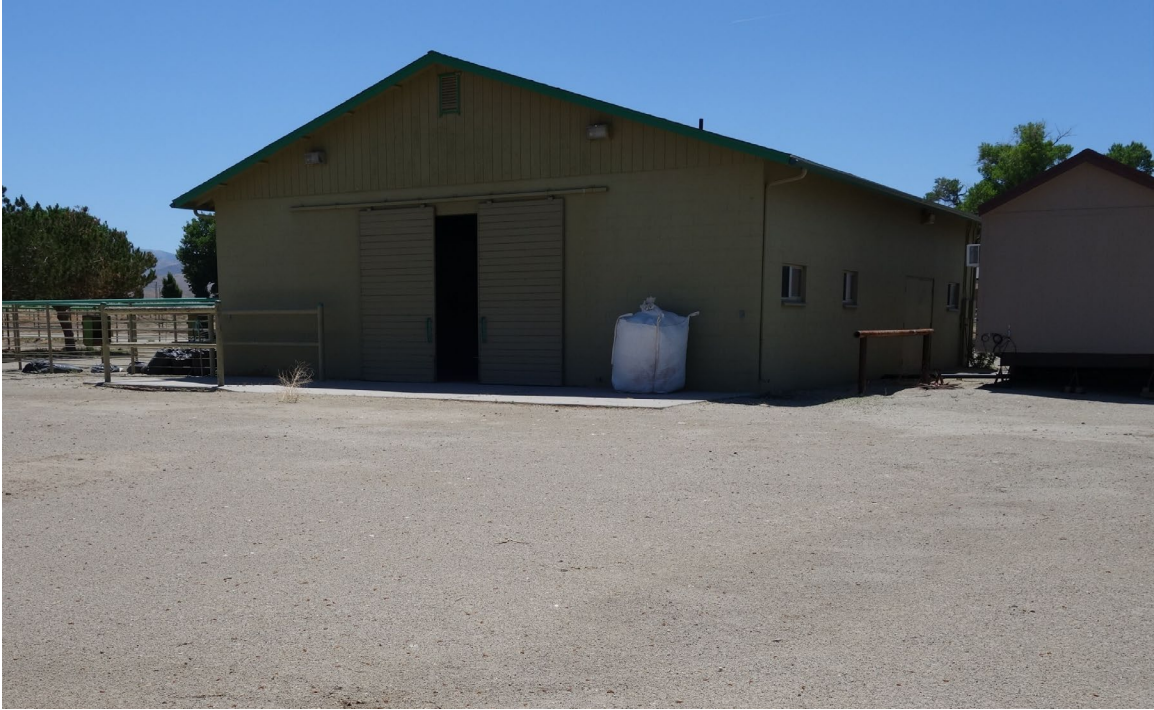
Horse Stable – FCA Building #3823 Description: Exterior of the Building.
