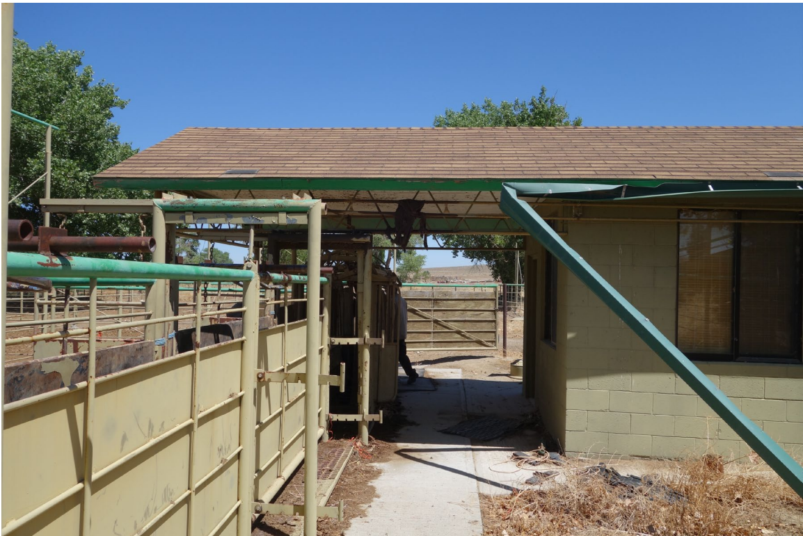
Veterinary Shed (Vacant) – FCA Building #3829 Description: Exterior of the Building.
