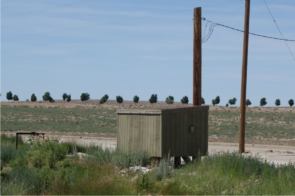
Pump House 1 – FCA Building #3835 Description: Exterior of the Structure.
