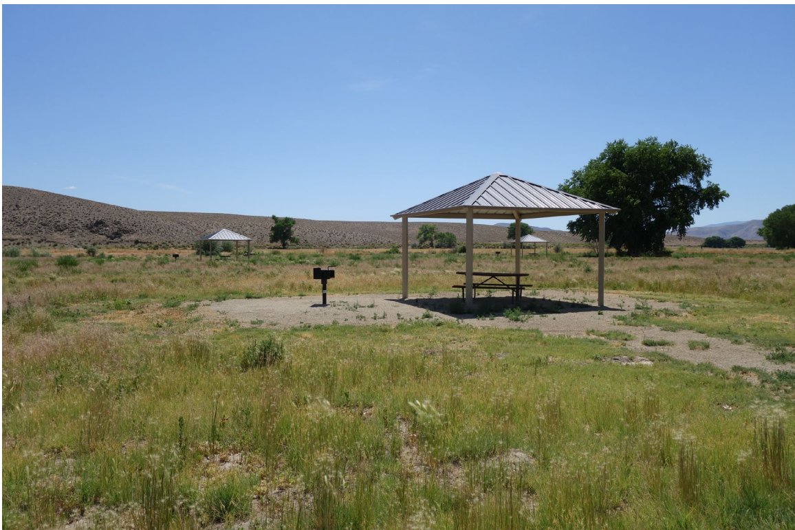
Ramada 23 through 26 – FCA Building #4052 through #4055 Description: Typical Shade Ramadas at Day Use Area.
