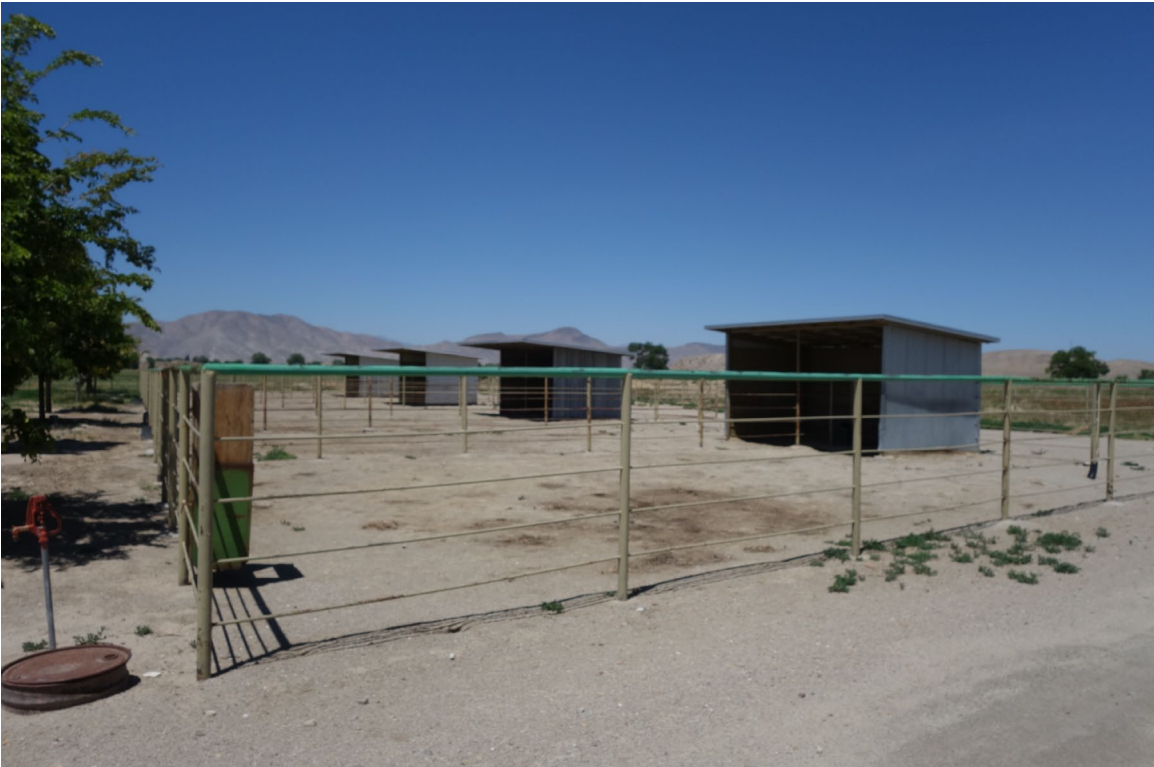
Metal Shed 1 through 4 – FCA Building #3831 through #3834 Description: Exterior of the Structures.
