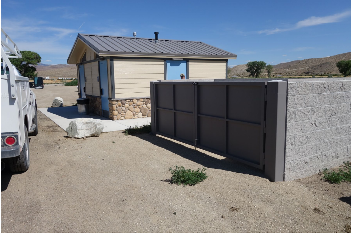
Comfort Station #4 – FCA Building #4051 Description: Exterior of the Building at Day Use Area.
