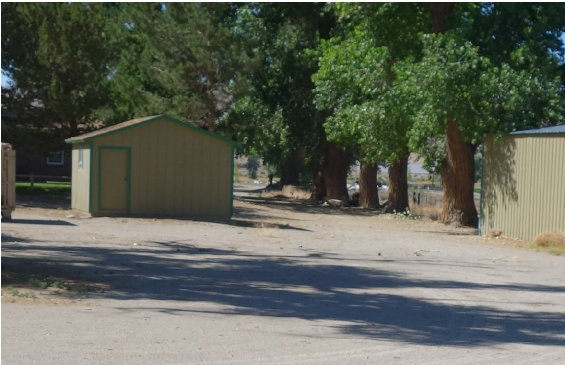
Pump House 2 – FCA Building #3836 Description: Exterior of the Building.
