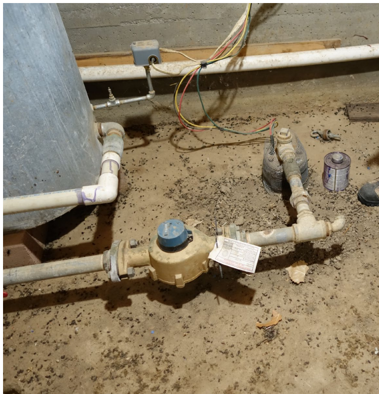
Bynum House Domestic Well Building – FCA Building #3821 Description: Well Refurbishment Recommended.
