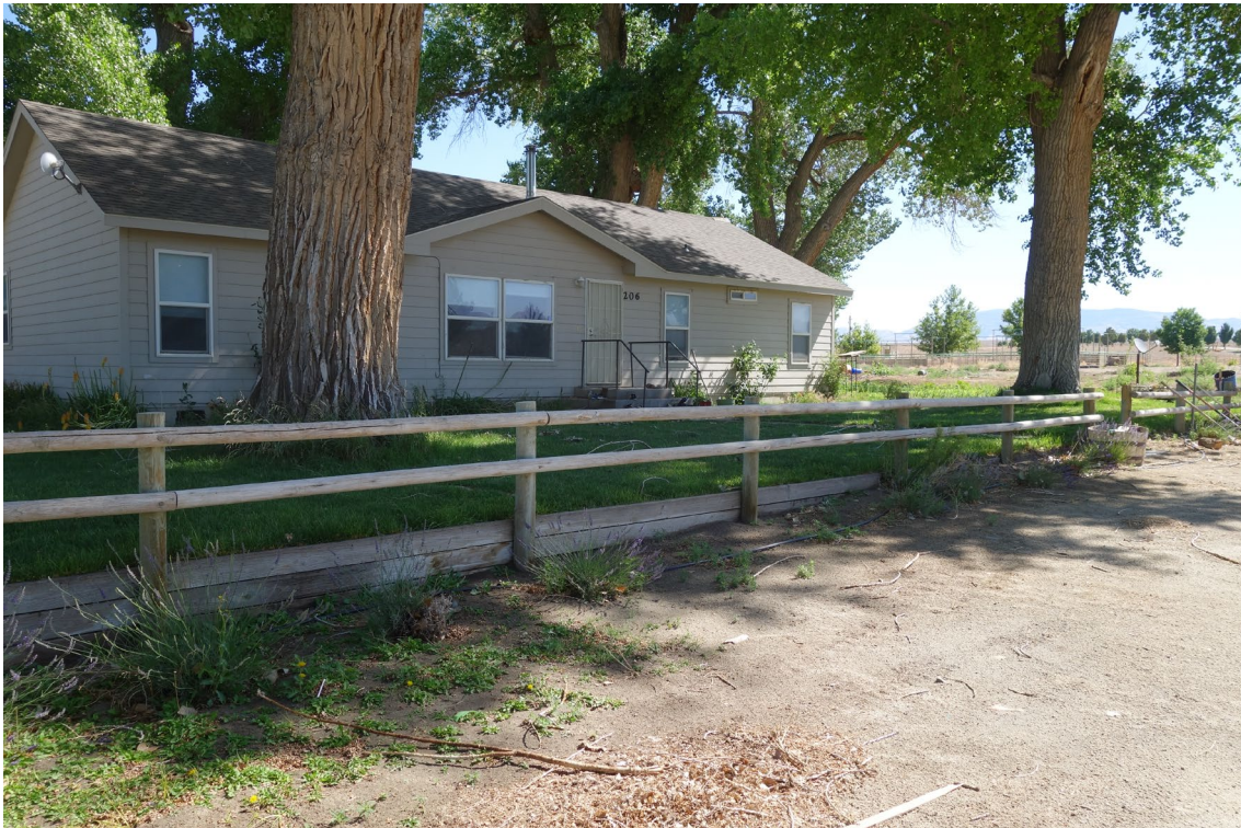
206 House - FCA Building #3814 Description: Exterior of the Building.
