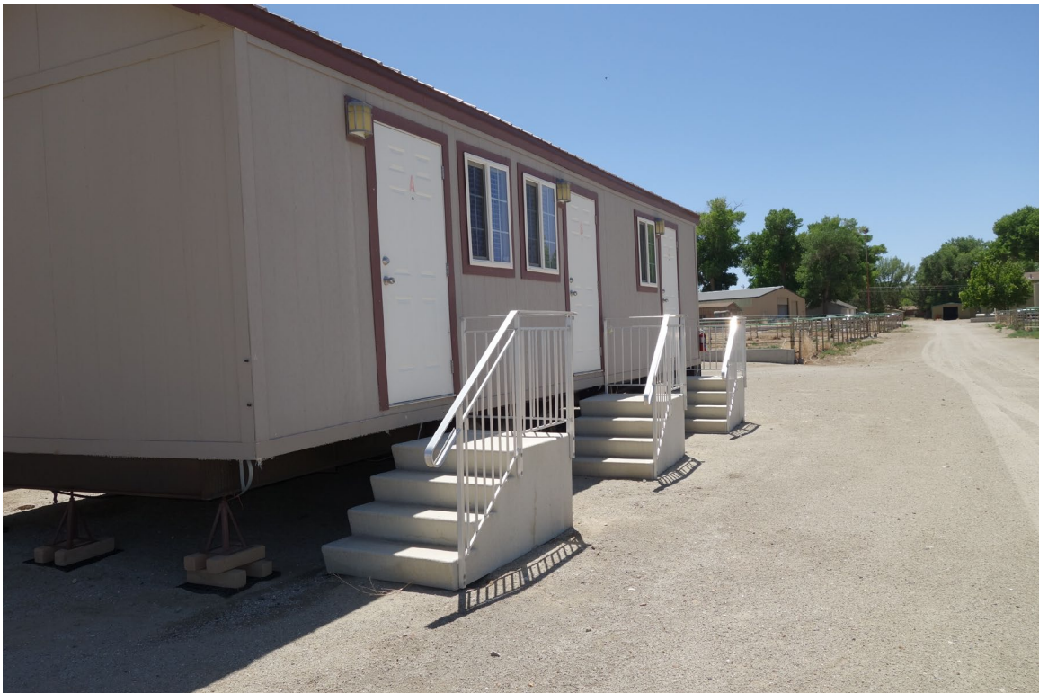
Man Camp Trailer #1 – FCA Building #4079 Description: Egress Door Landing Adjustment.
