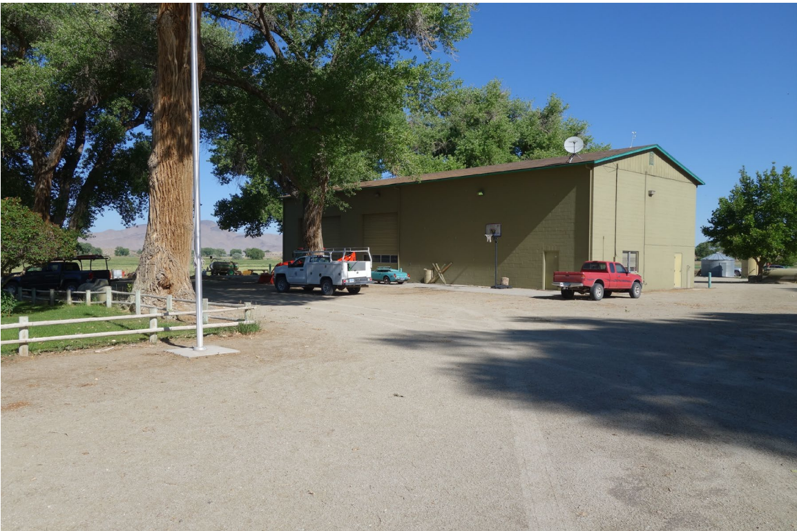
Park Maintenance Shop – FCA Building #3824 Description: Exterior of the Building.
