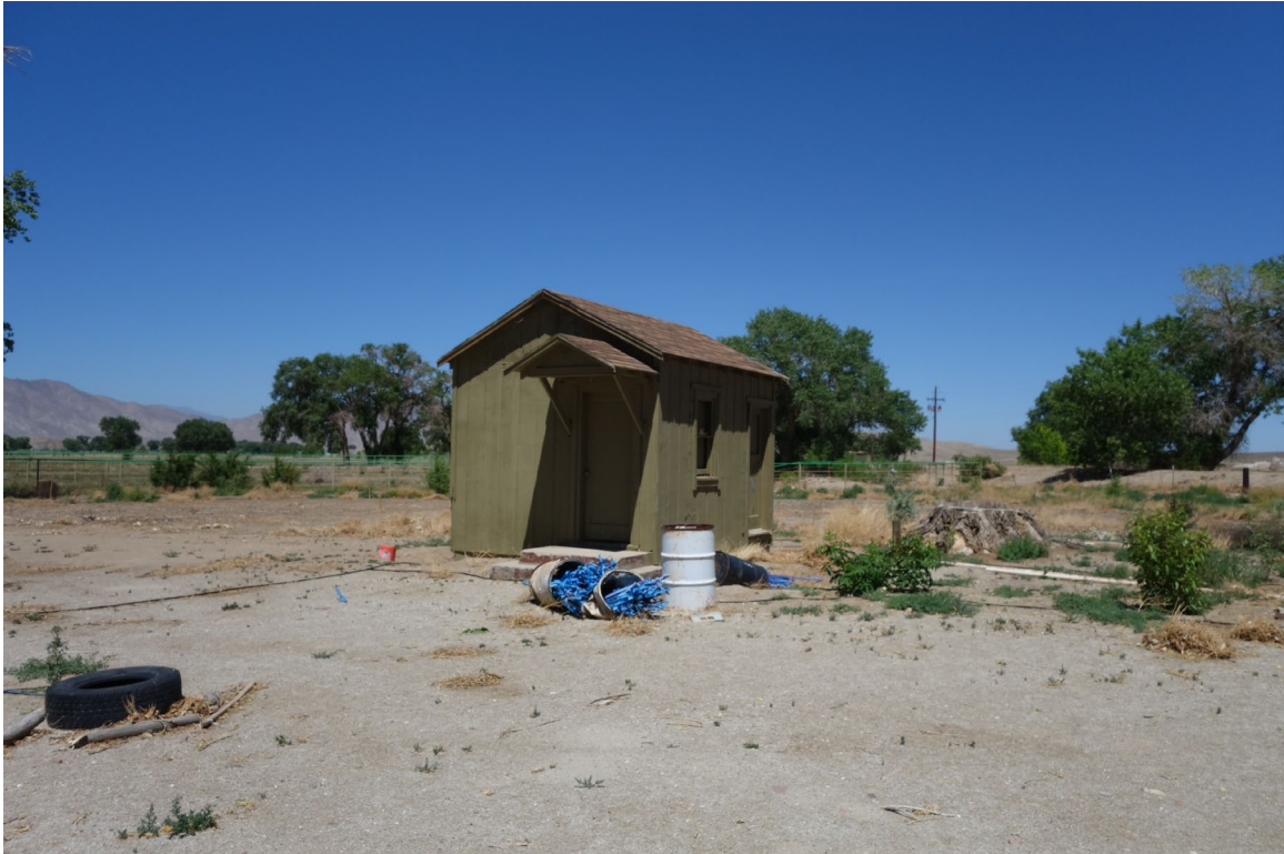
Bynum House Domestic Well Building – FCA Building #3821 Description: Exterior of the Building.
