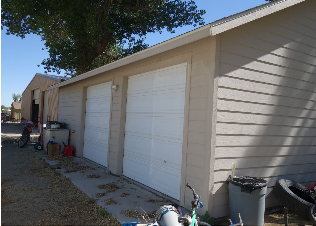
206 House Detached Garage – FCA Building #3815 Description: Exterior of the Building.
