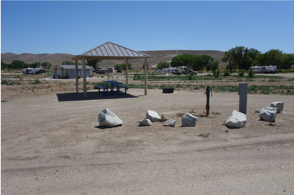
Ramada 27 through 49 – FCA Building #4056 through #4078 Description: Typical Shade Ramadas at Quail Run RV Camping Area.
