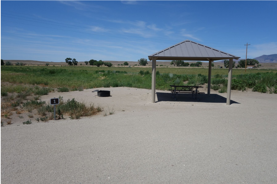
Ramada 1 through 16 – FCA Building #3880 through #3895 Description: Typical Shade Ramadas at Primitive Camping Area.
