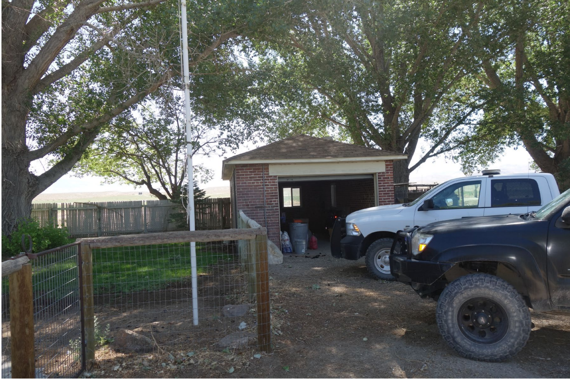
Brick House Detached Garage – FCA Building #3817 Description: Exterior of the Building.
