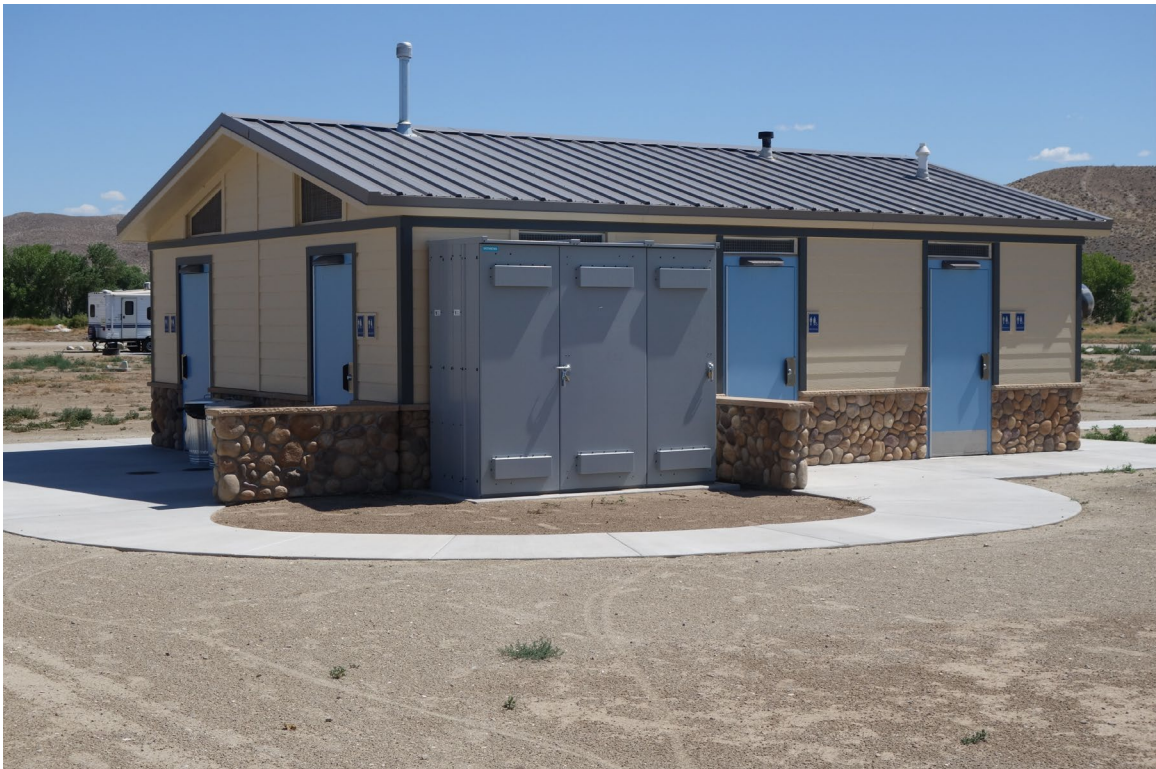
Comfort Station #3 – FCA Building #4050 Description: Exterior of the Building at Quail Run RV Camping Area.
