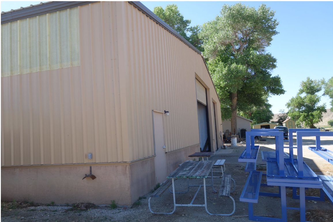
Broad Shed – FCA Building #3827 Description: Exterior of the Building.
