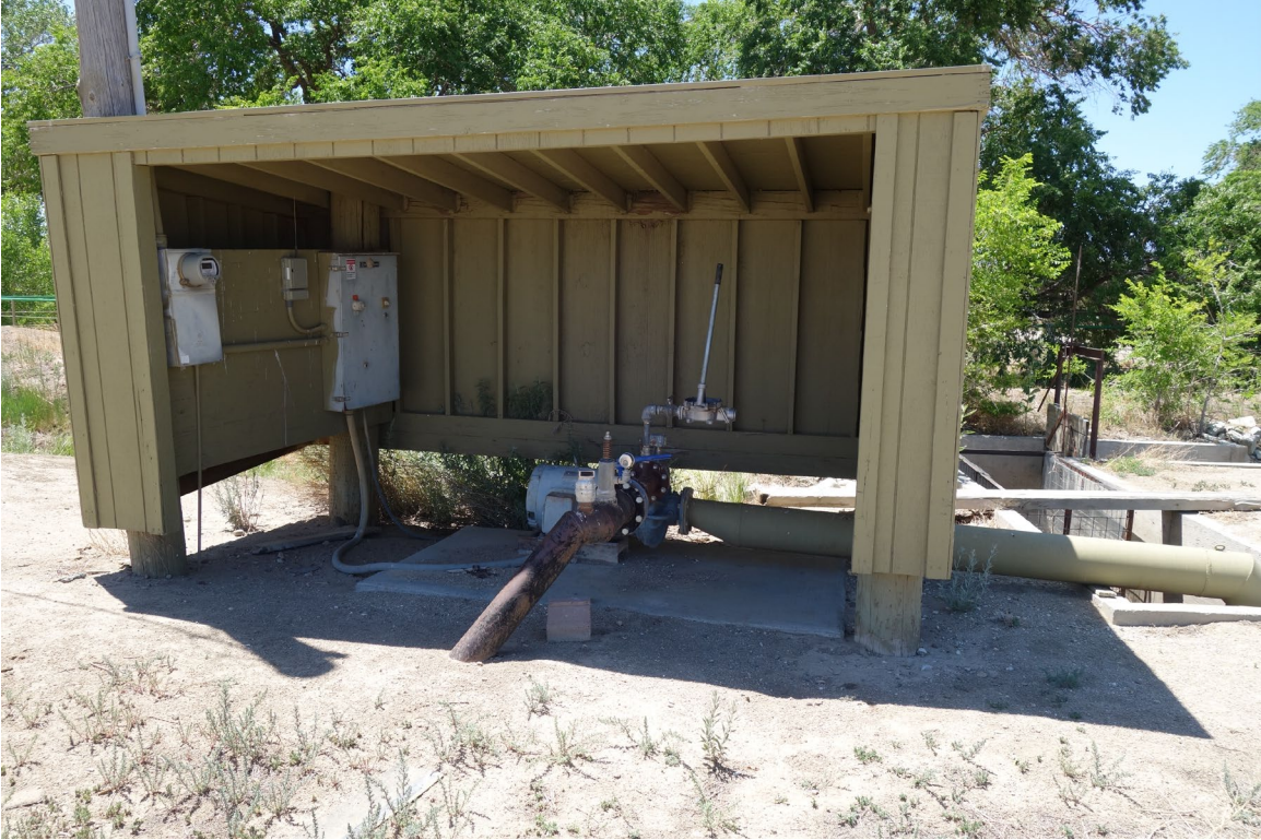
Pump House 3 – FCA Building #3837 Description: View of the Structure.
