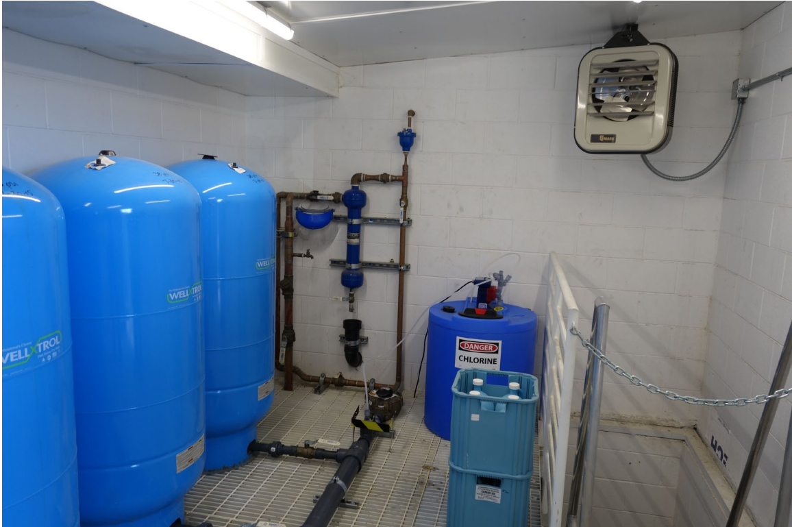
Guest House Domestic Well Building – FCA Building #3819 Description: Interior of the Building.
