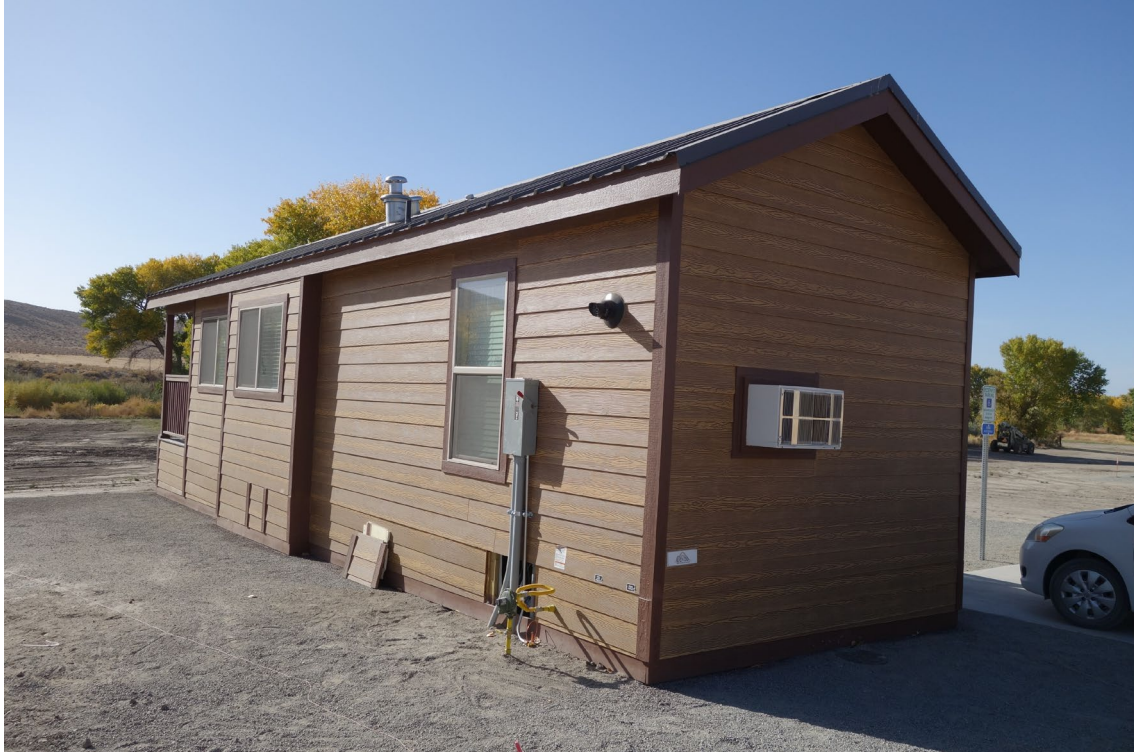
Cabins #1 - #5 – FCA Building #4104, 4105 & 4149, 4150 Description: View of Typical Cabin.
