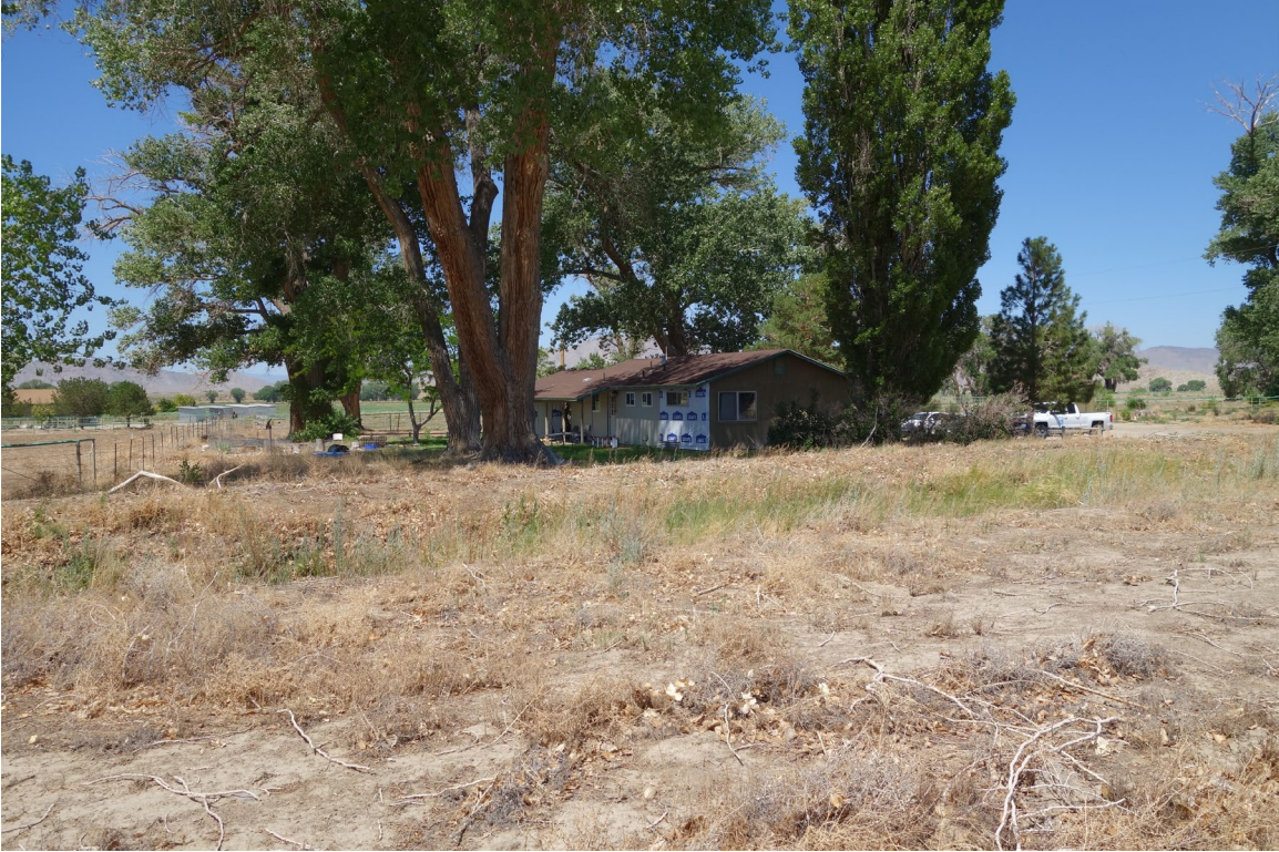
Bynum House – FCA Building #3820 Description: Exterior of the Building.
